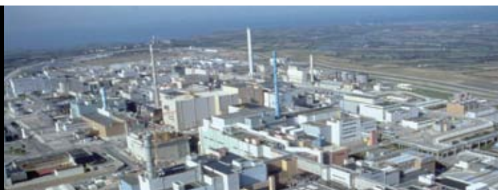
Overall view of La Hague reprocessing plant.
